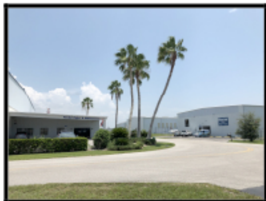
New Naples Offices and Hangar
